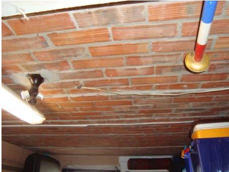
NeHoBo-vloeren in souterrain
