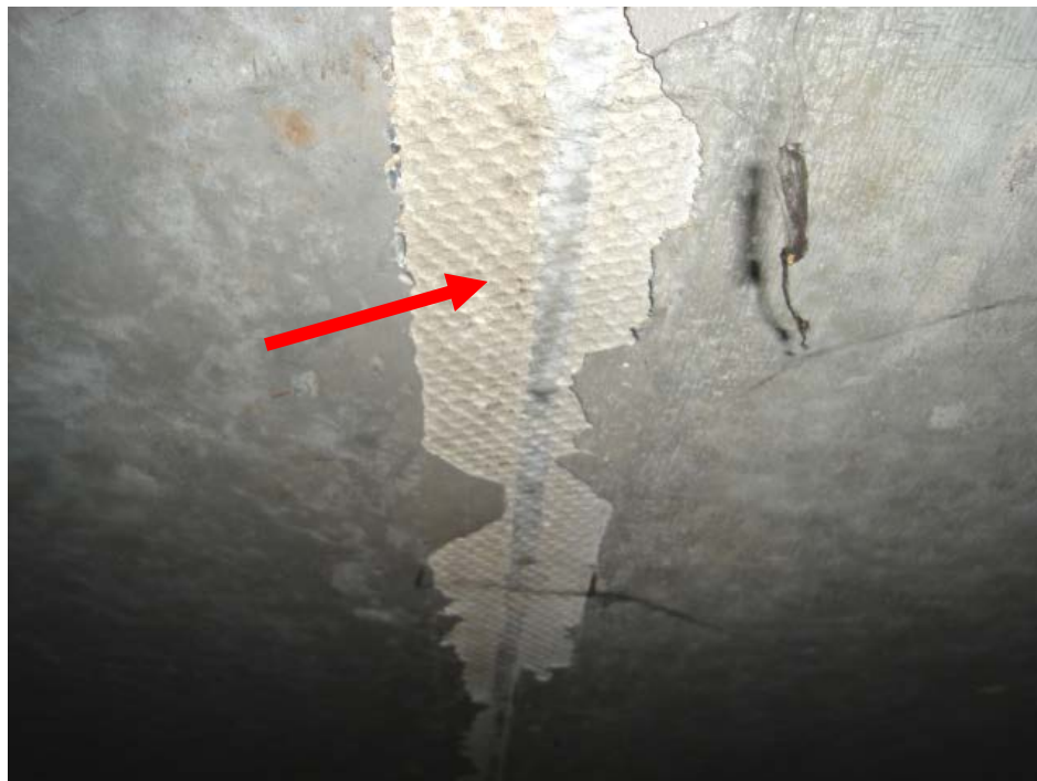
foto: 24, verloren bekisting (cement)
